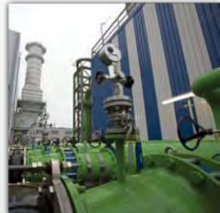
Process Control Timer for Irrigation Pumps
