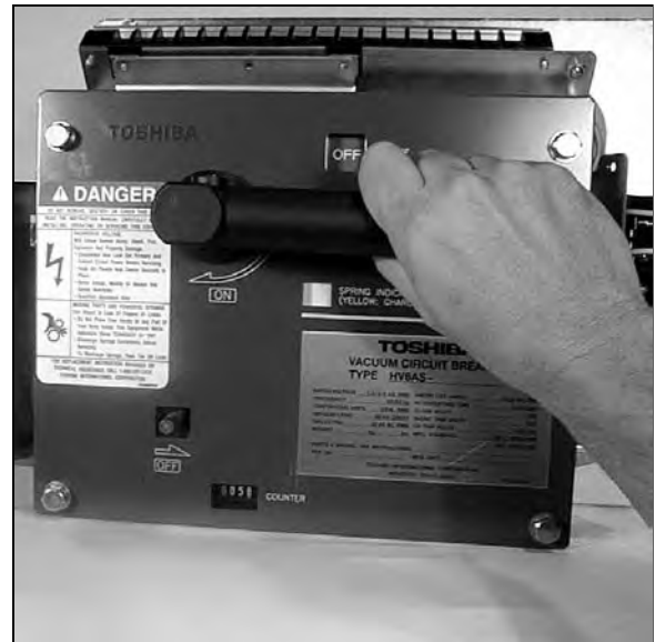
Fig. 23 Preparing to Manually Close Breaker
